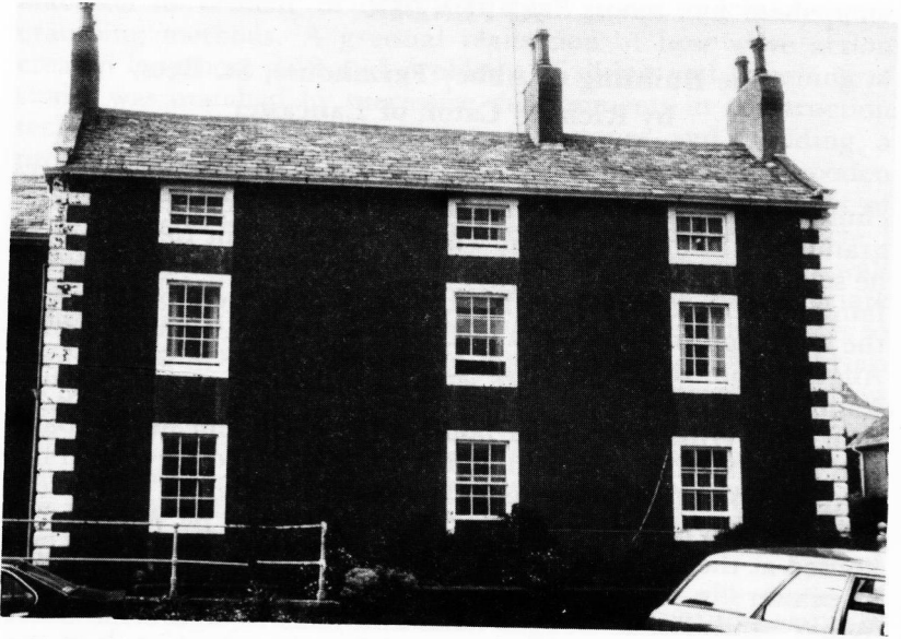
Abbey Farmhouse, St. Bees. (a) Southeast elevation painted dark brown. (b) Northeast gable with dated doorway.
